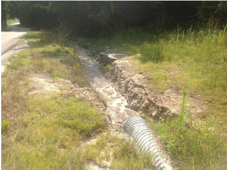
Bedrock outcrop on existing KY 1442
